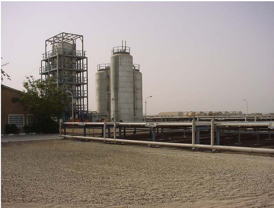
Figure 1. Picture of Abu Dhabi solar desalination plant.
